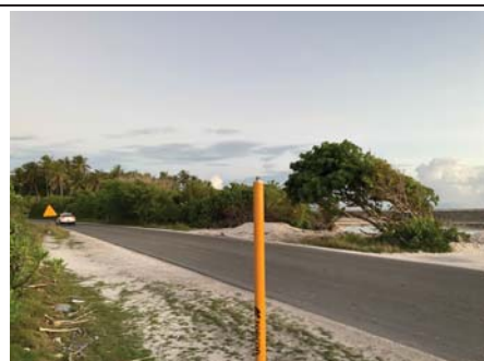
Height 1.3m SOUTH VIEW Distance 2m
